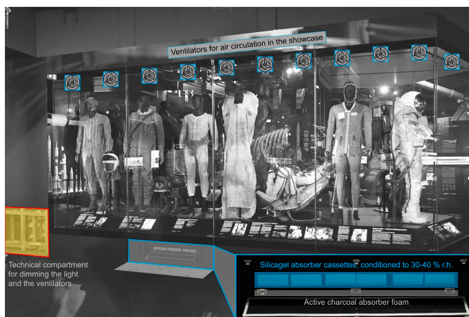
Figure 3. Absorbent materials in the showcase drawers to remove pollutants from the atmosphere (grey) and to buffer relative humidity (blue). See also the detail on the right. Control unit for the ventilators and dimming light on the left (yellow).
